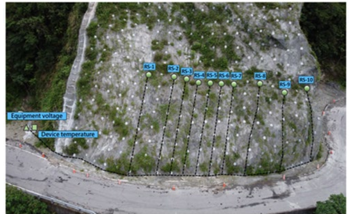
Fig 6 West Side Rock bolt stress sensor (stress gauge): 10 sets
